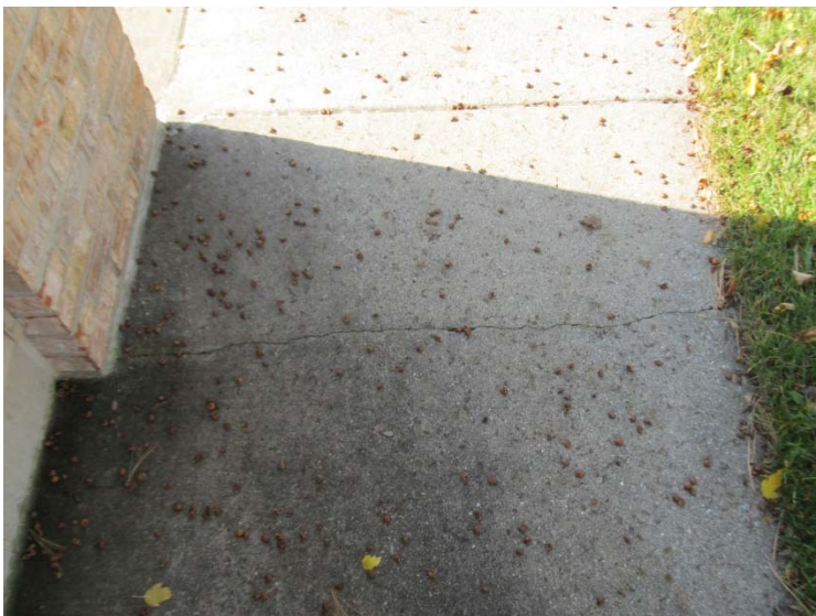
Sidewalk crack at 3518 Kirkaldy Circle
