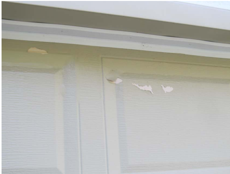
Finish deterioration at 3662 Tartan Circle
