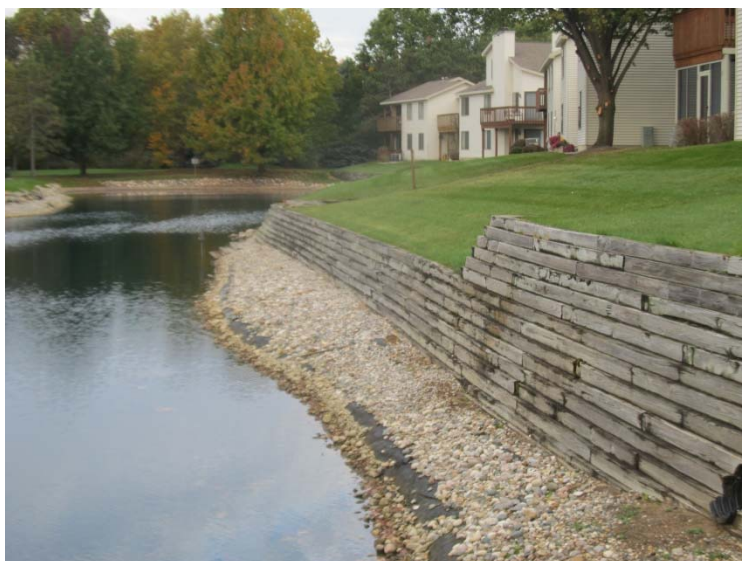
Timber retaining wall overview
