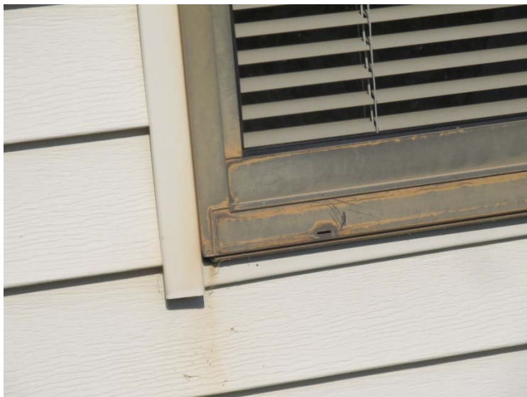
Window frame deterioration at 3770 Tartan Circle
