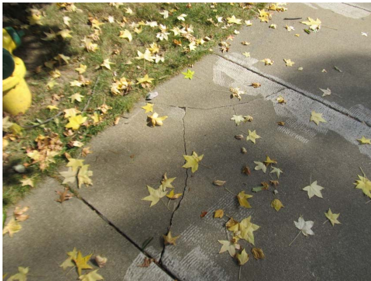
Sidewalk Cracks
