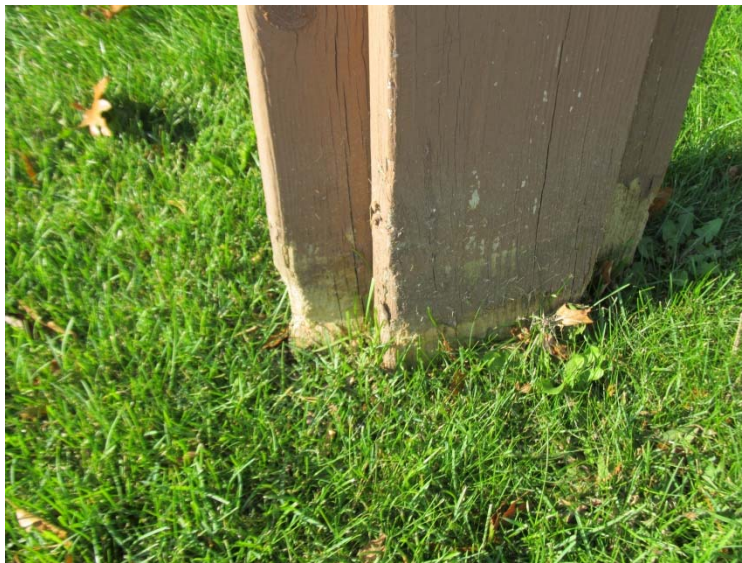
Wood deterioration at light pole
