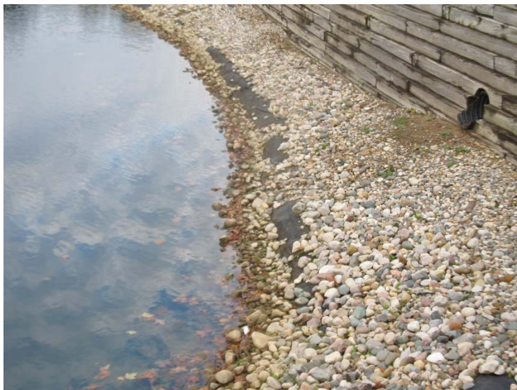
Loss of stone rip rap at south pond
