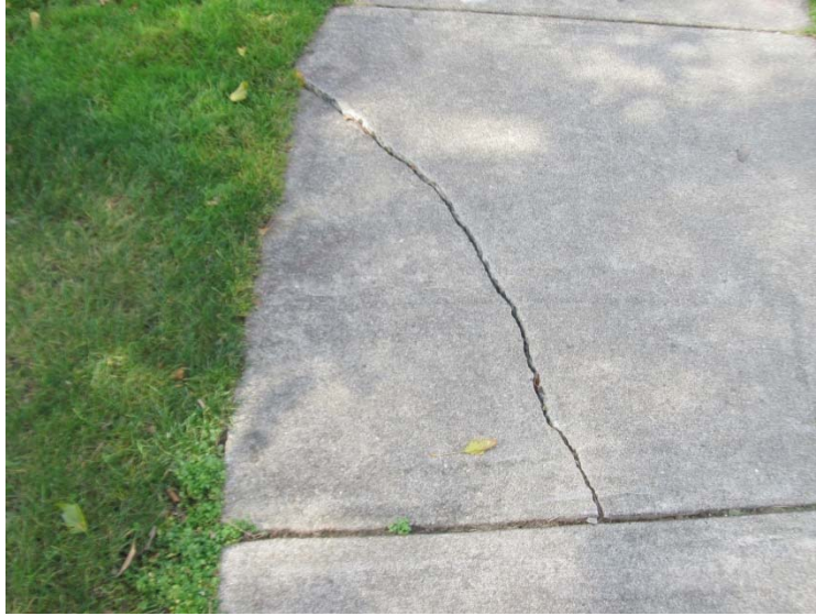
Sidewalk crack
