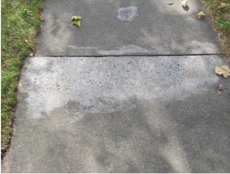
Spalled concrete
