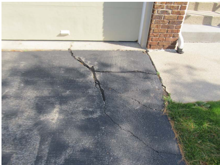
Driveway cracks at 3601 Tartan Circle
